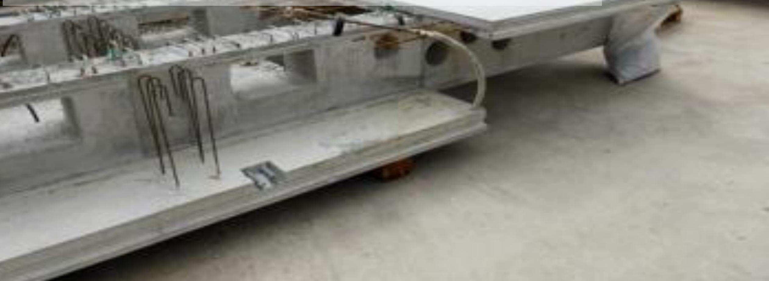
**Precast elements:** more than structural concrete but spiked with all kinds of pipes, tubes and terminal devices for the building service
