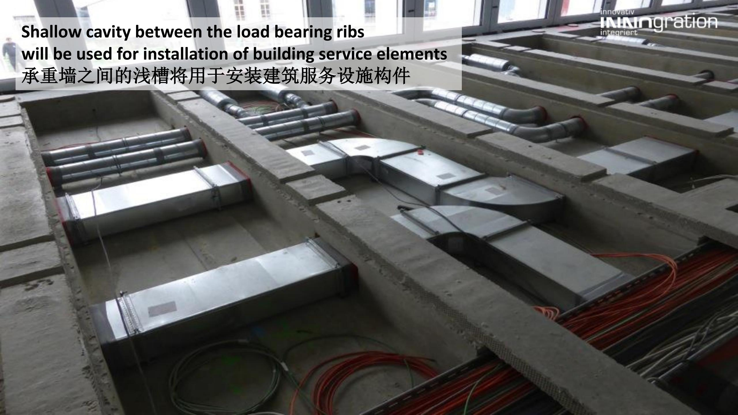
Shallow cavity between the load bearing ribs and openings
