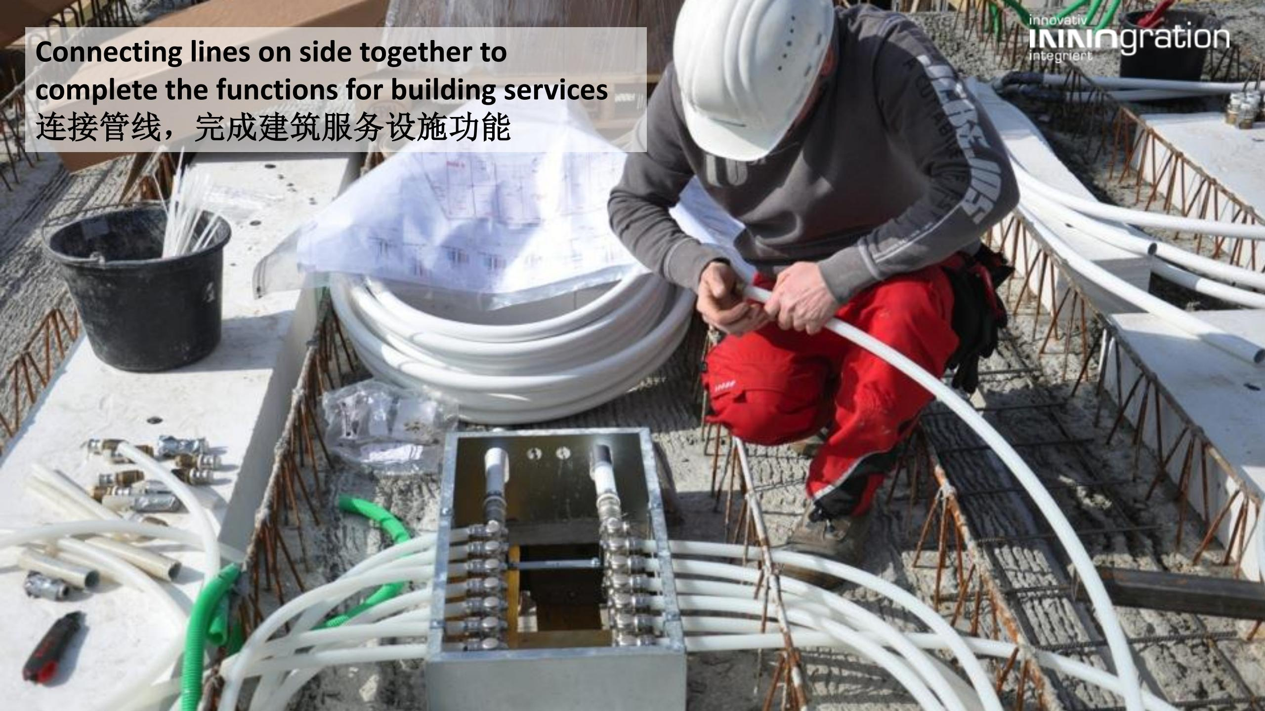
**Shallow cavity between the load bearing ribs is used for the preassembled heat distributor in order to organize heating and cooling with thermoactive component system**
