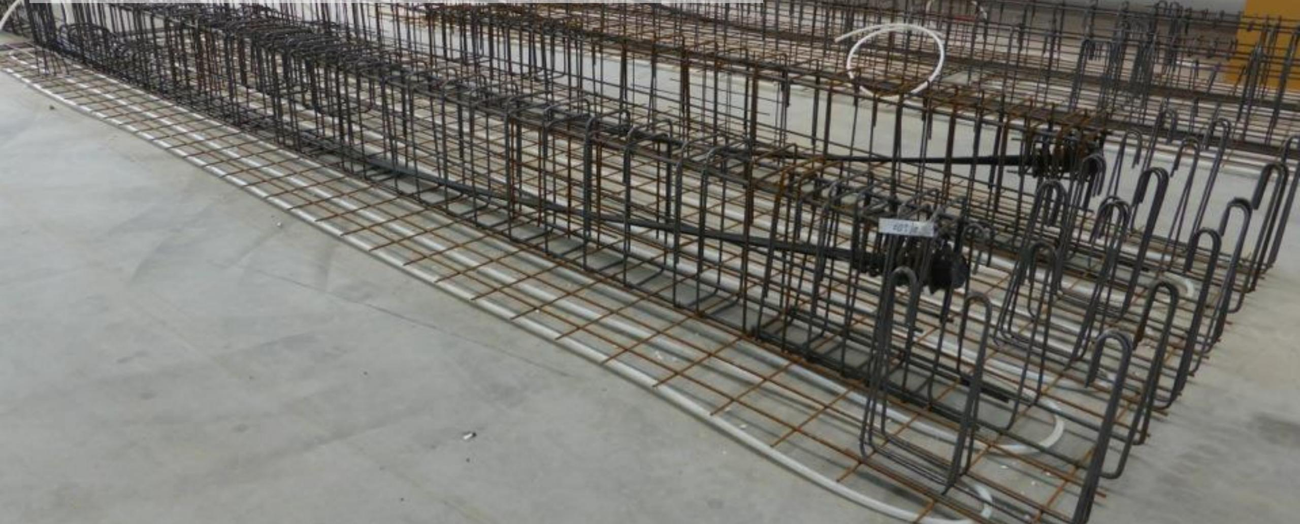
Shallow cavity and large opening in the load bearing ribs allows tubes and pipes to be placed in each direction
