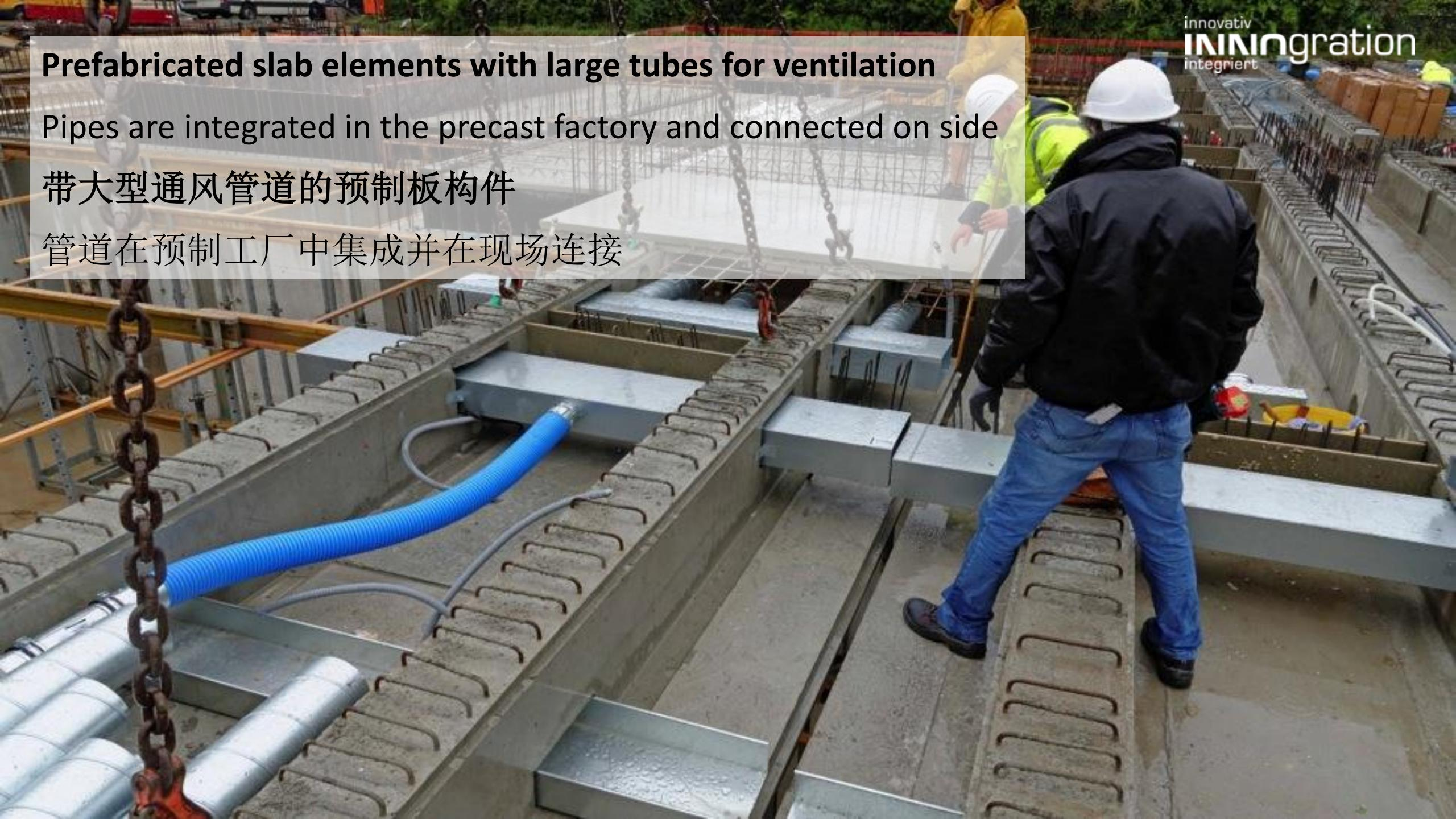
**Shallow cavity between the load bearing ribs
