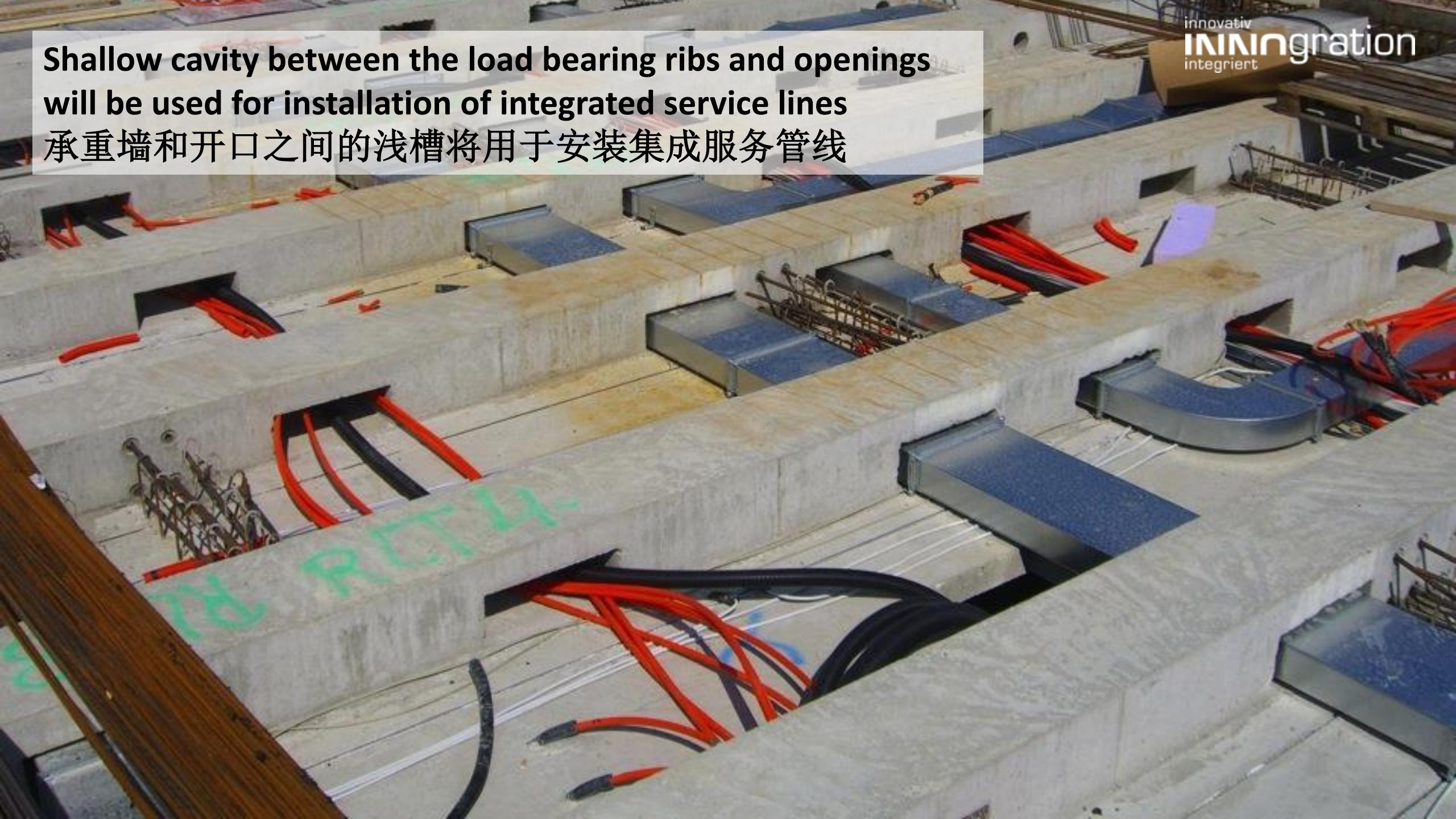
Connecting lines on side together to complete the functions for building services
