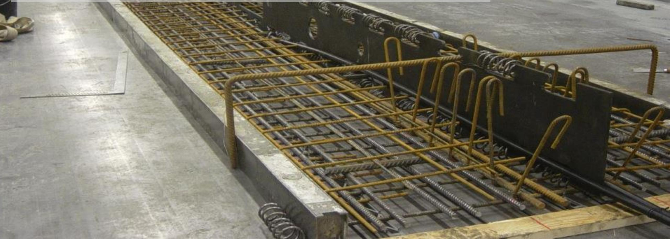
**Structural elements with multiple options for the installation of building service (HVACR) devices Prestressing devices and tubes for heating/cooling**
